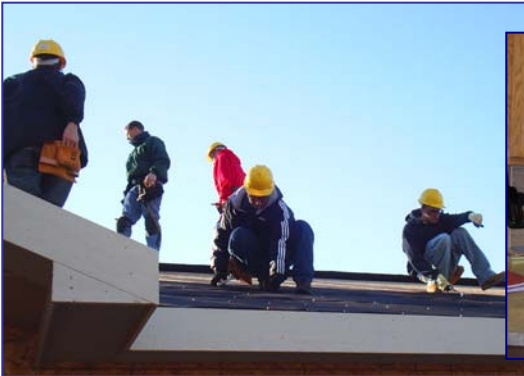
Top left: Contractors replace a roof.
